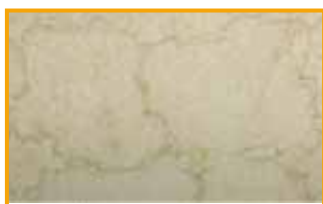
Marbling caused by impurities in steam condensate
