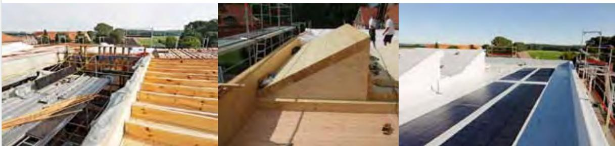
HOLZ II - DACH MIT TAFEL- UND MASSIVHOLZELEMENTEN
