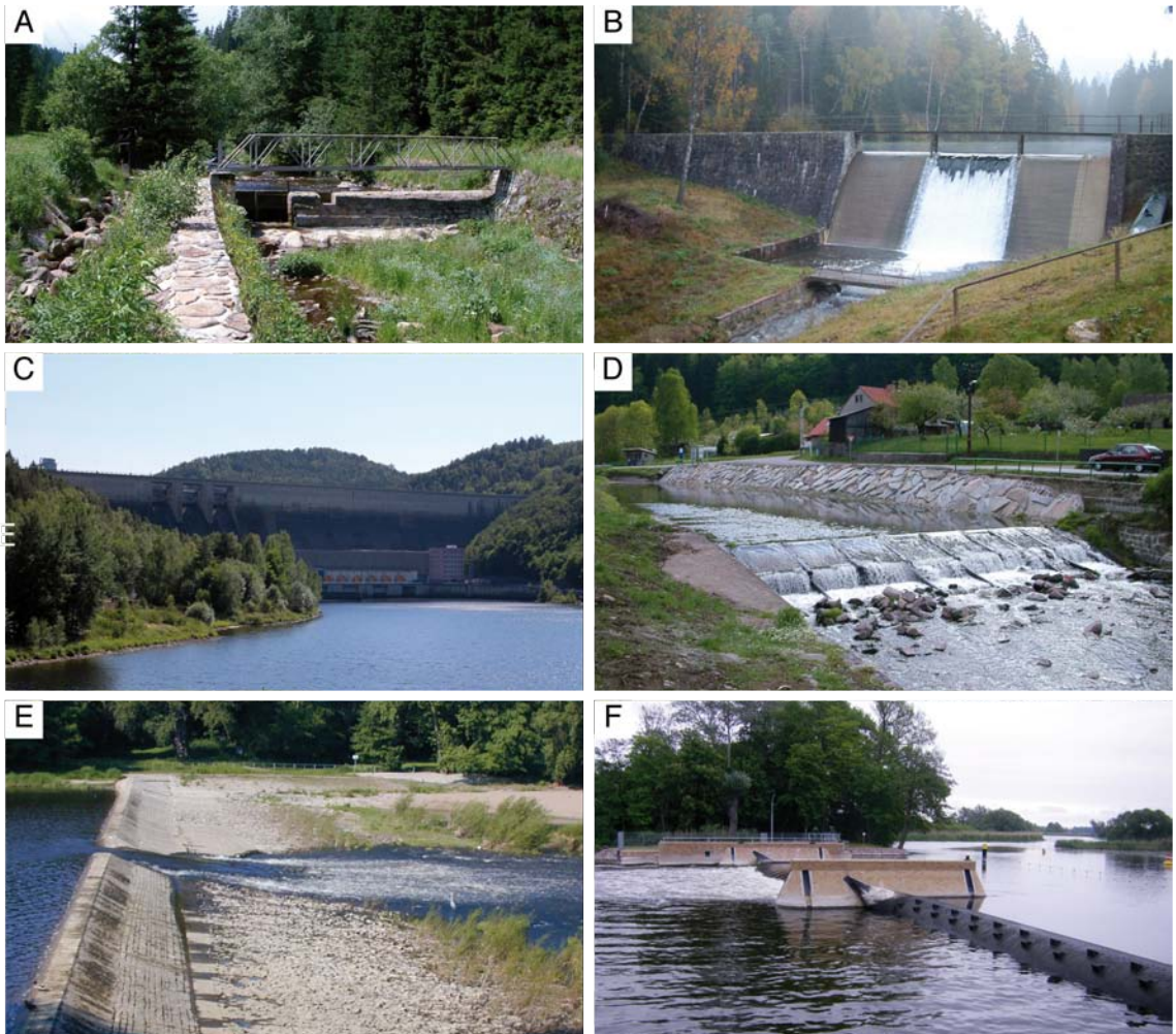
Figure 1. Examples of different types of barriers in the River Elbe network: (A) small weir Františkov in the upper River Vltava, equipped with a non-functional fish pass. (B) small dam Černé jezero in the River Úhlava, no fish pass. (C) large Orlík dam in the River Vltava, highest dam (91 m) in the Czech Republic, no fish pass. (D) weir Čenkov in the River Litavka, no fish pass. (E) weir in the river branch Alte Elbe at Magdeburg. (F) weir in the River Havel at Bahnitz, equipped with a fish pass.
