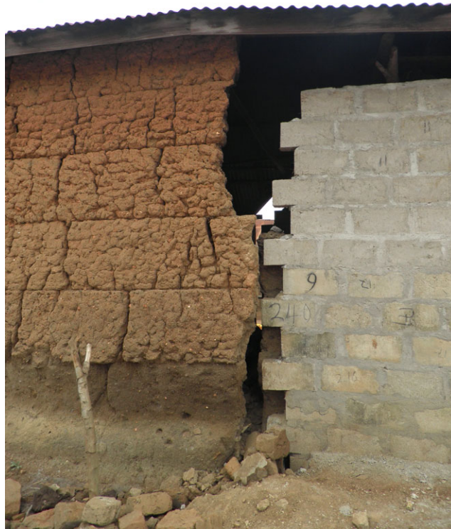
FIGURE 2 A house being renovated with income from cashew.
