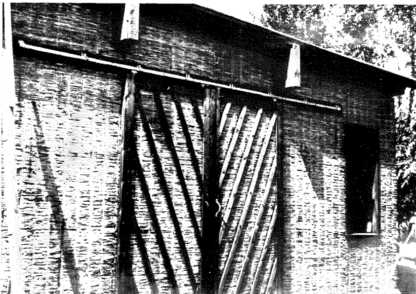
Figure 15. Shed constructed from reed boards.
