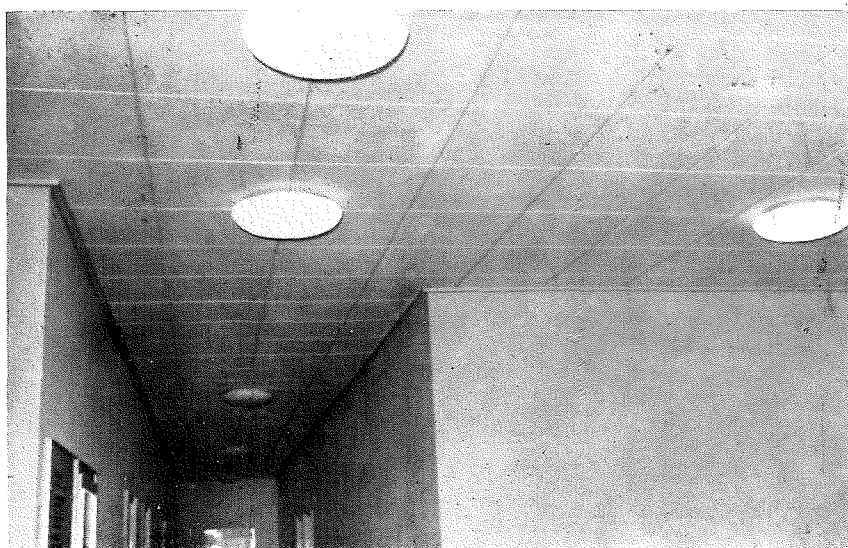
Figure 9. Waste board ceiling with decorative grooves.
