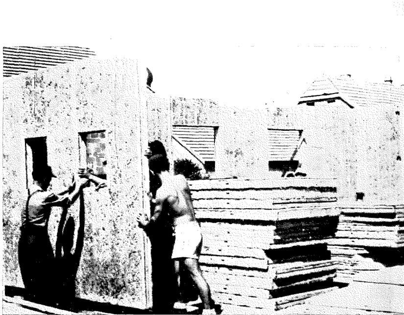
Figure 10. Utilization of mineralized wood-wool slabs for low-cost houses.
