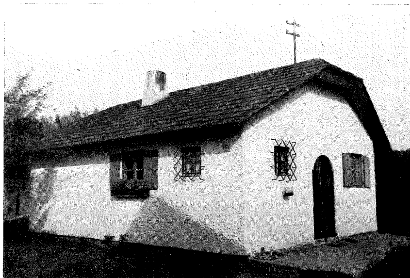
Figure 8. Bungalow built from waste boards (cement coating).
