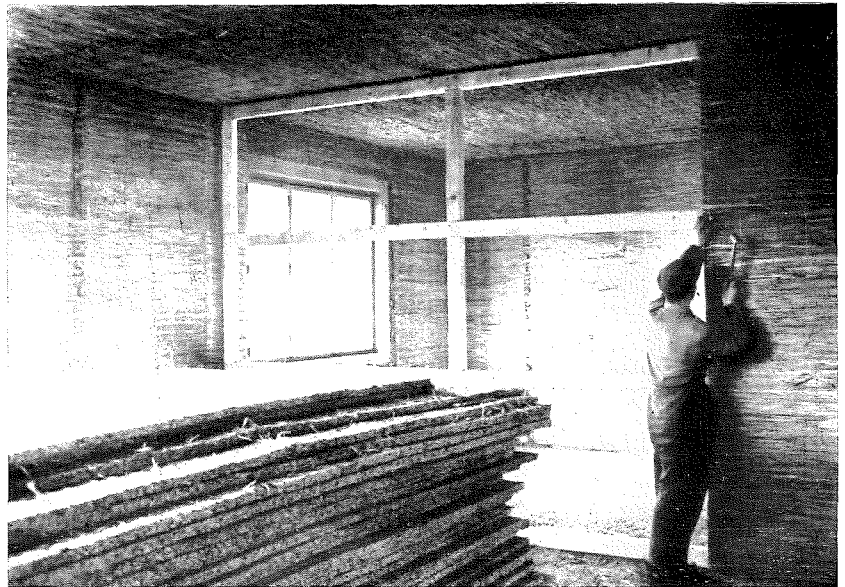
Figure 14. Mounting reed boards in a building.
